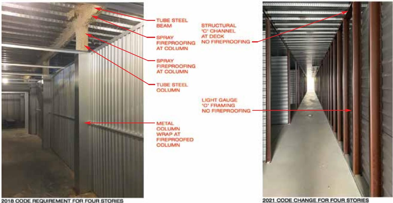
Changes to the 2021 International Building Code increased the height of sprinklered self storage facilities from three stories to four stories, for buildings made of Type IIB materials (unprotected steel) and Type IIIB materials (noncombustible or fire-retardant-treated wood stud exterior walls and any interior construction). Image: Jeffrey S. Dallenbach, AIA, Managing Partner of San Antonio, Texas-based DALLENBACH • COLE ARCHITECTURE (formerly Archcon Architecture)
